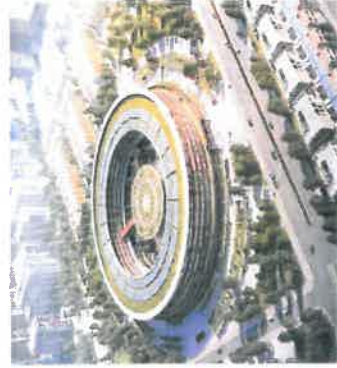
The EDGE-certified FPT Complex in Danang, Vietnam.
