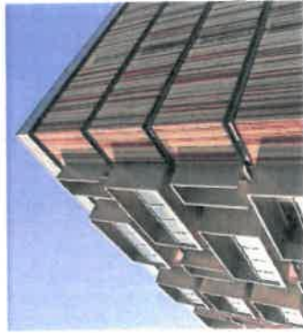
Located in Changping, the Passive House "Bruck" by Landsea has ambitions to become EDGE-certified.
