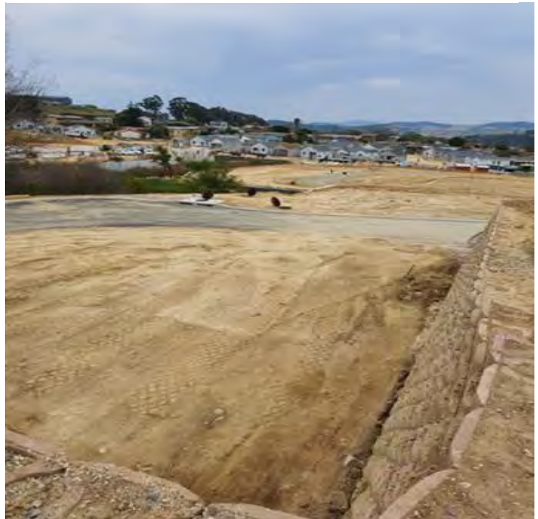
Figure 3:13: Installation of services complete
