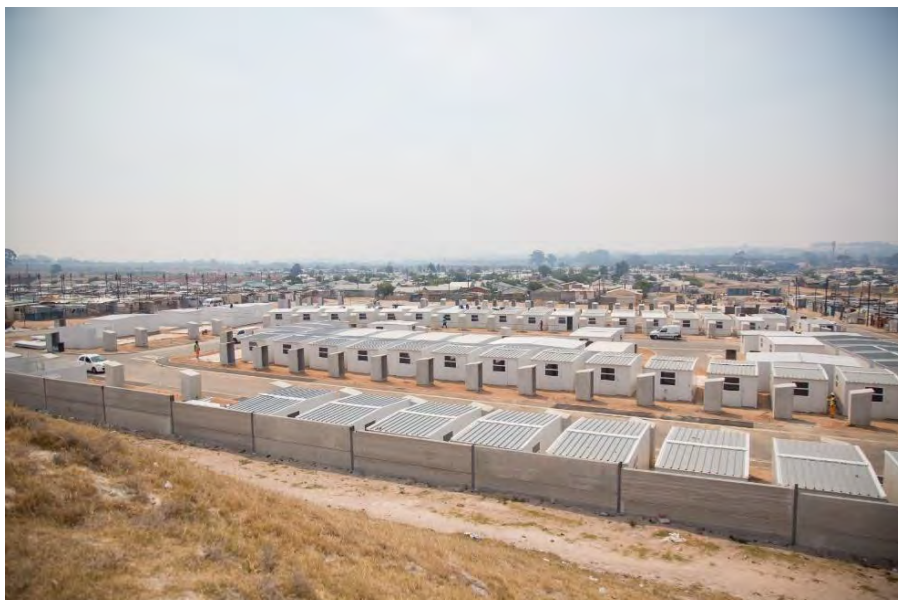
Completion of construction of TRA
