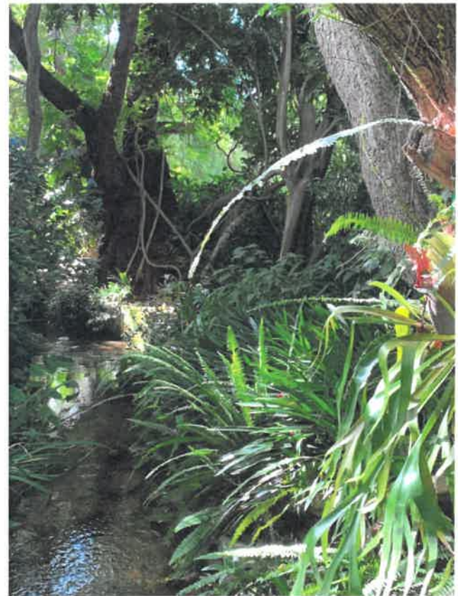
TREES AND OVERHANG ON NORTHERN BANK.
