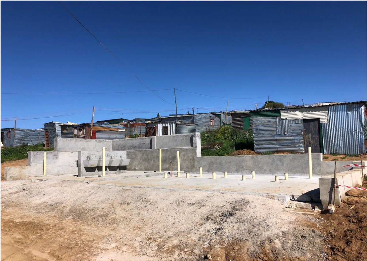
Figure 37: Construction of basic services, Watergang Informal Settlement
