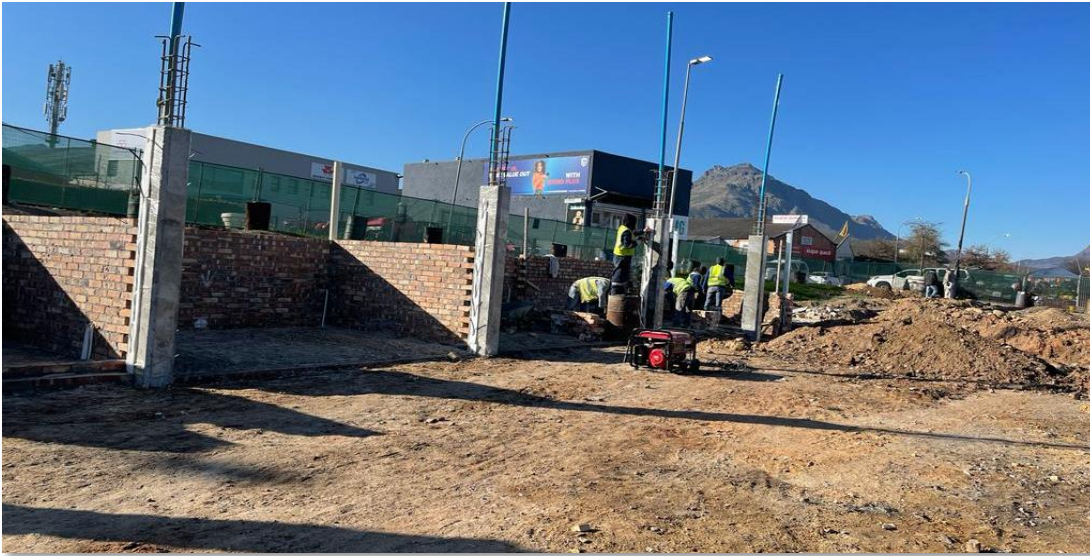
Figure 43: Construction of new taxi rank (Bird Street)
