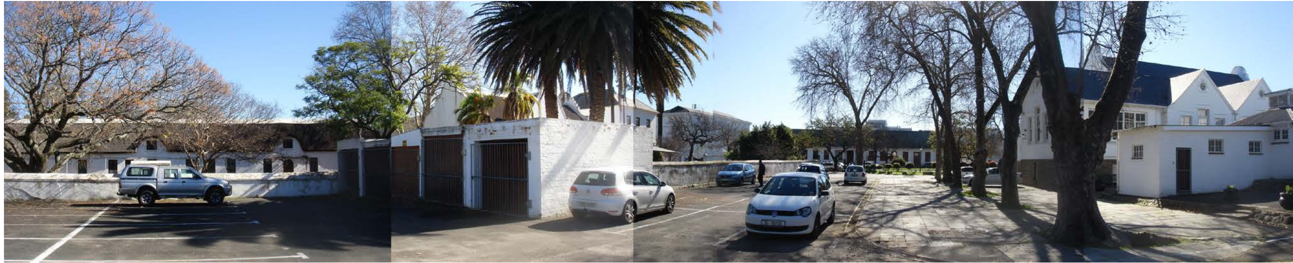
Figure 21: View of parking garages separating current parking area spaces behind Rhenish School and Institute buildings.
