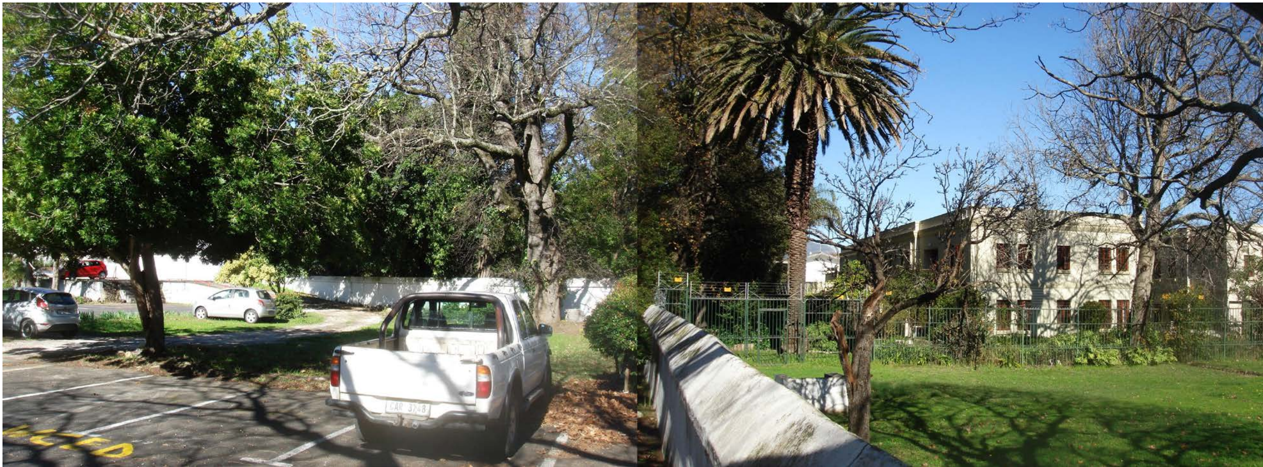
Figure 25: View of wall separating Rhenish lower terrace carpark and area behind the Rhenish Parsonage looking south.
