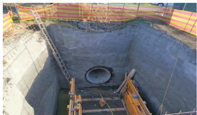
Figure 41: Sewer Crossing Bottelary Road (Devonbosch)
