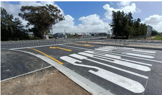
Figure 42: Klapmuts Road intersection Upgrade
