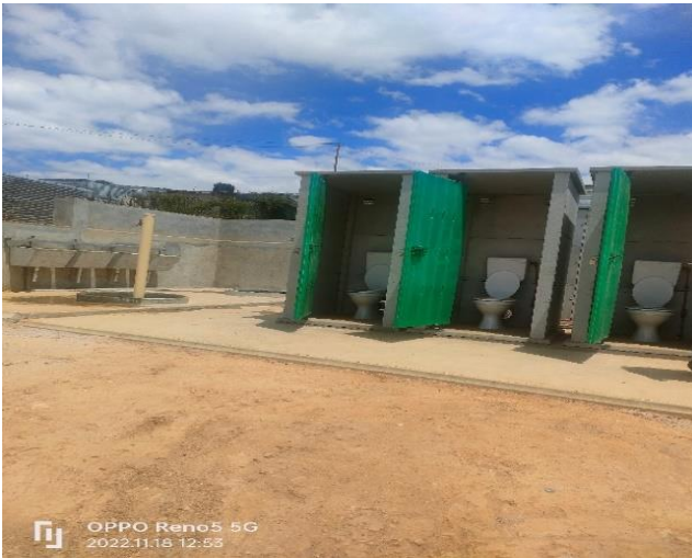
Figure 36: Construction of basic services, Watergang Informal Settlement
