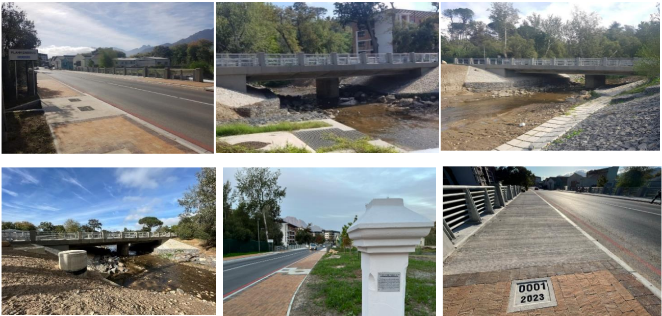
Figure 32: New Bridge constructed
