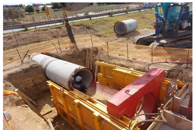
Figure 47: Outfall Sewer upgrade (Newinbosch)
