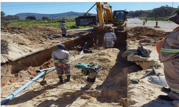
Figure 44: Cloeteville Bulk water upgrade (Voliere)
