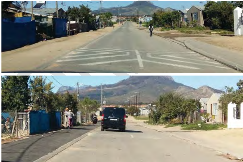
Photo's 11 and 12 - Before and after Adams Road Klapmuts – surfaced left hand side sidewalk
