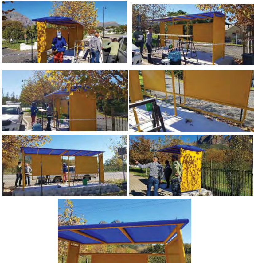
2 No. shelters installed in Pniel Main road near the church.
