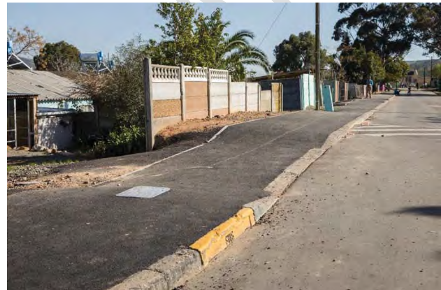
Photo 18 – Eike Street upgrade Cloeteville
