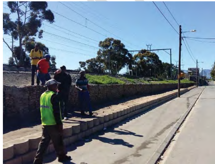
Photo's 15 and 16 Before and after at Beyers Street sidewalk
