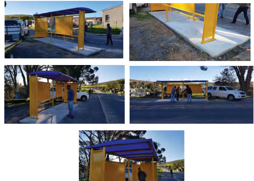
1 No. shelter installed in Cloetesville in Lang street just Outside "SmartieTown".
