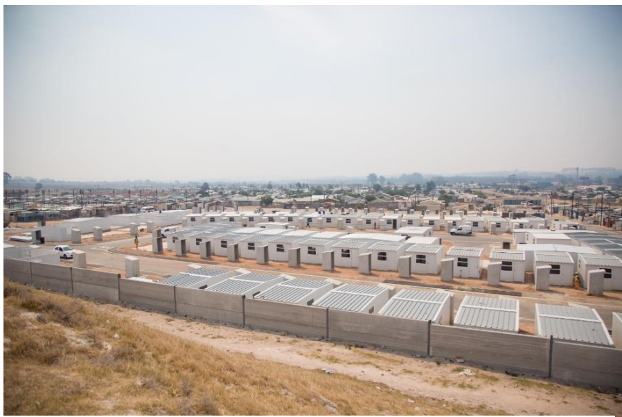
Completion of construction of TRA
