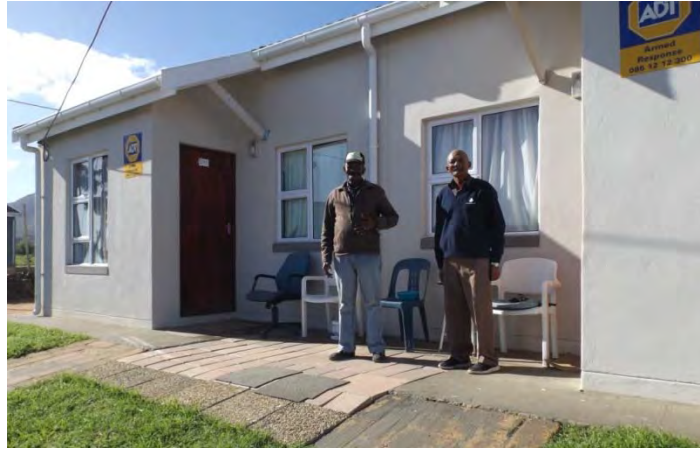
Figure 52 Families from the Blaauwklippen community re-located to the new development
