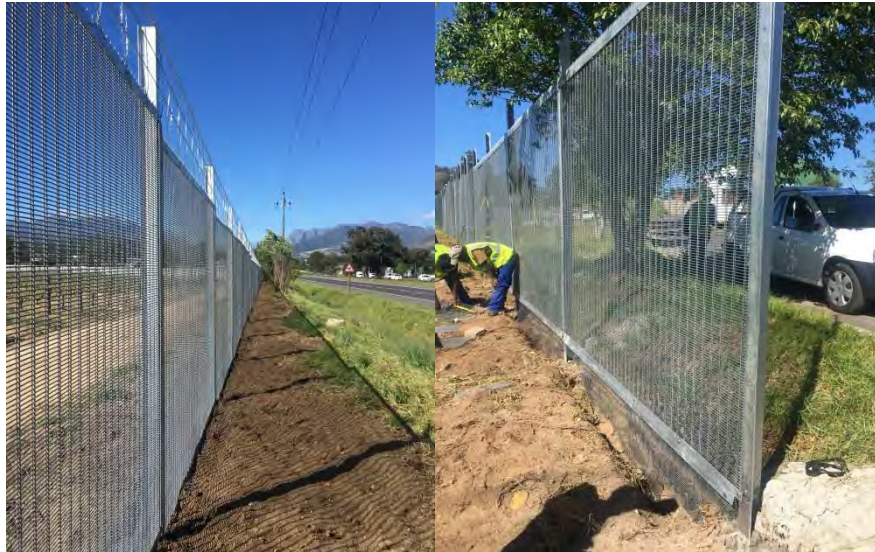
Figure 35 Fence installation at DVLS (ASARA)
