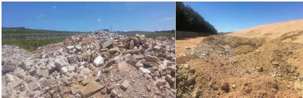
Figure 16 Uncrushed rubble stockpiled on site
