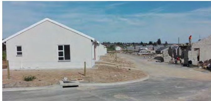
Figure 51 Construction in process
