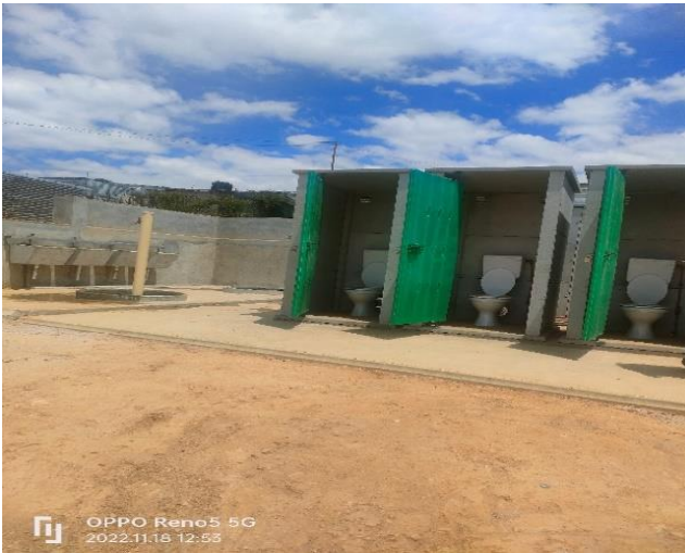
Figure 36: Construction of basic services, Watergang Informal Settlement
