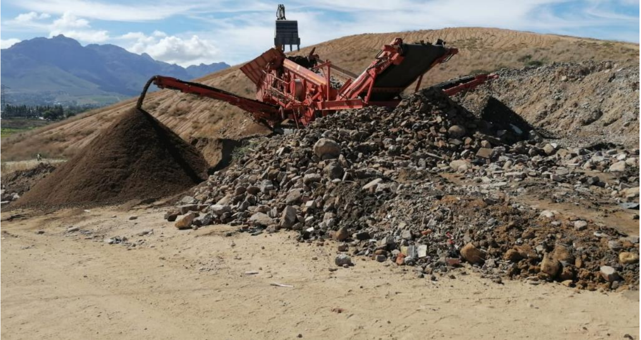
Figure 16: Crushing of builders rubble done on site
