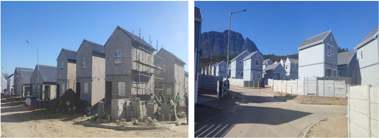
Figure 34: GAP Housing Project
