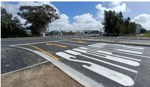
Figure 42: Klapmuts Road intersection Upgrade
