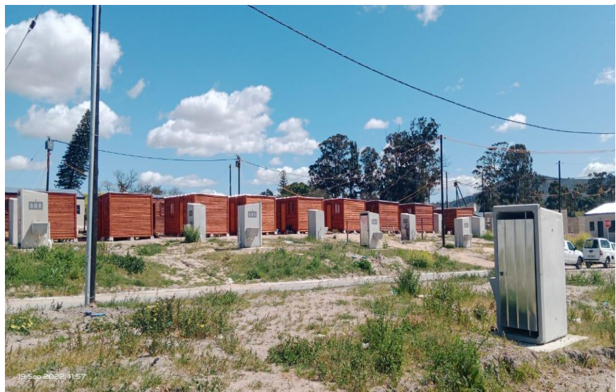
Figure 26: The temporary relocation units (wendy houses) with access to basic services
