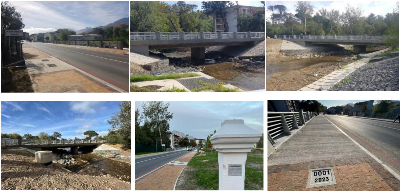
Figure 32: New Bridge constructed
