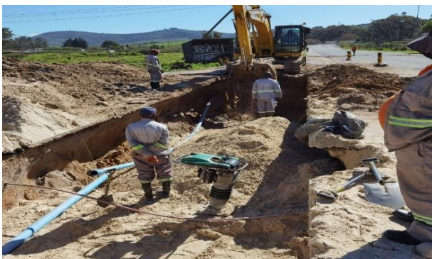
Figure 44: Cloetesville Bulk water upgrade (Voliere)
