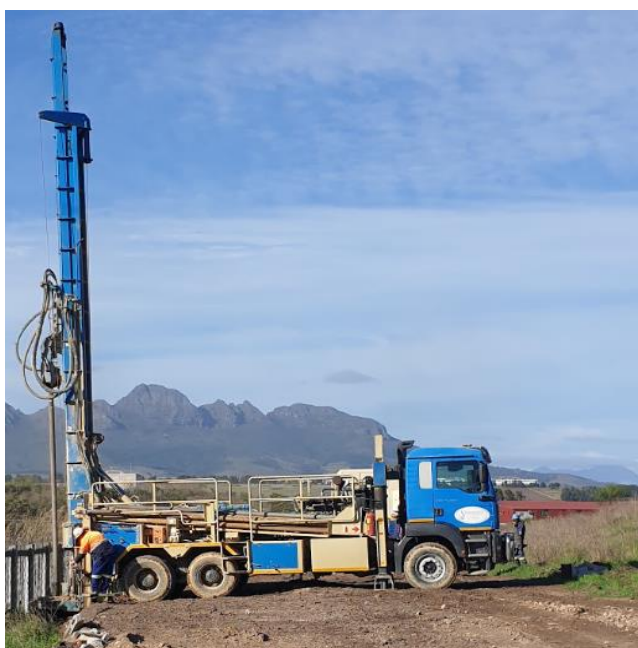
Photo: Drilling of well on-site
