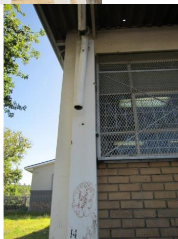
Figure 30 Broken light
