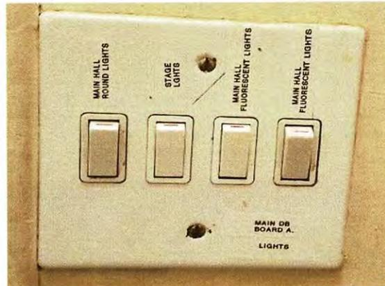
Fig. 10 Indication Full Labelling of Emergency Exit Light Fittings and Light Switches
