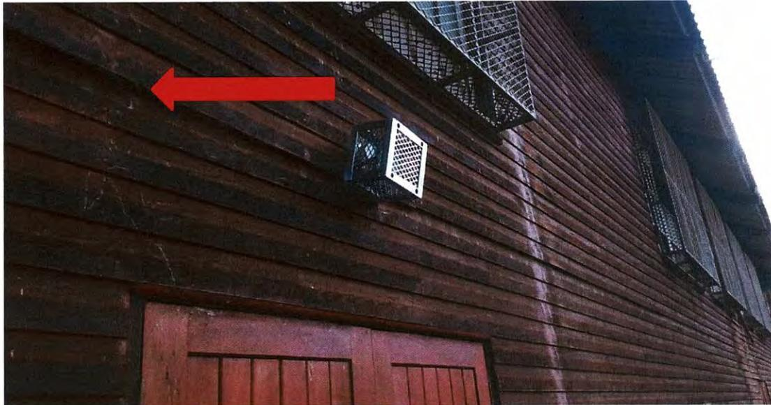
Fig. 6 All Exterior Flood fittings and Day Night Switch – Supply cable hidden under Wooden Fascia Boards
