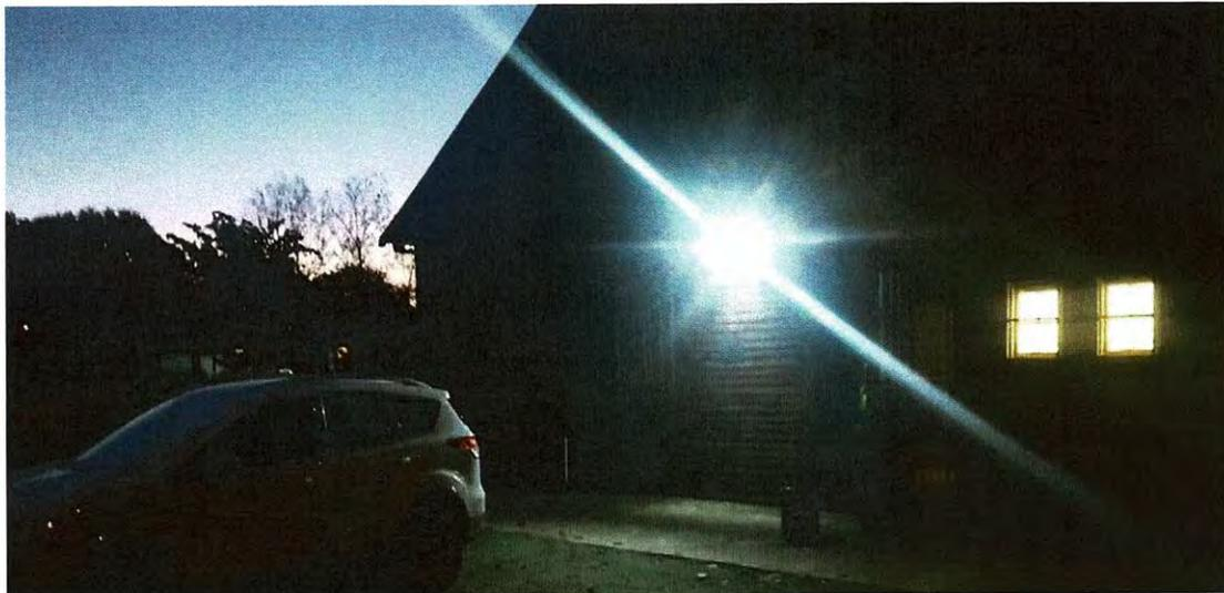
Fig. 8 Night Testing of All Exterior Flood lights – Power Switched Off
