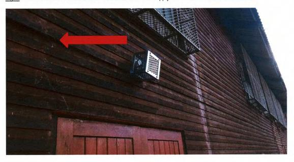
Fig. 6 All Exterior Flood fittings and Day Night Switch - Supply cable hidden under Wooden Fascia Boards
