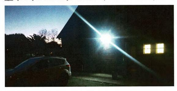
Fig. 8 Night Testing of All Exterior Flood lights - Power Switched Off
