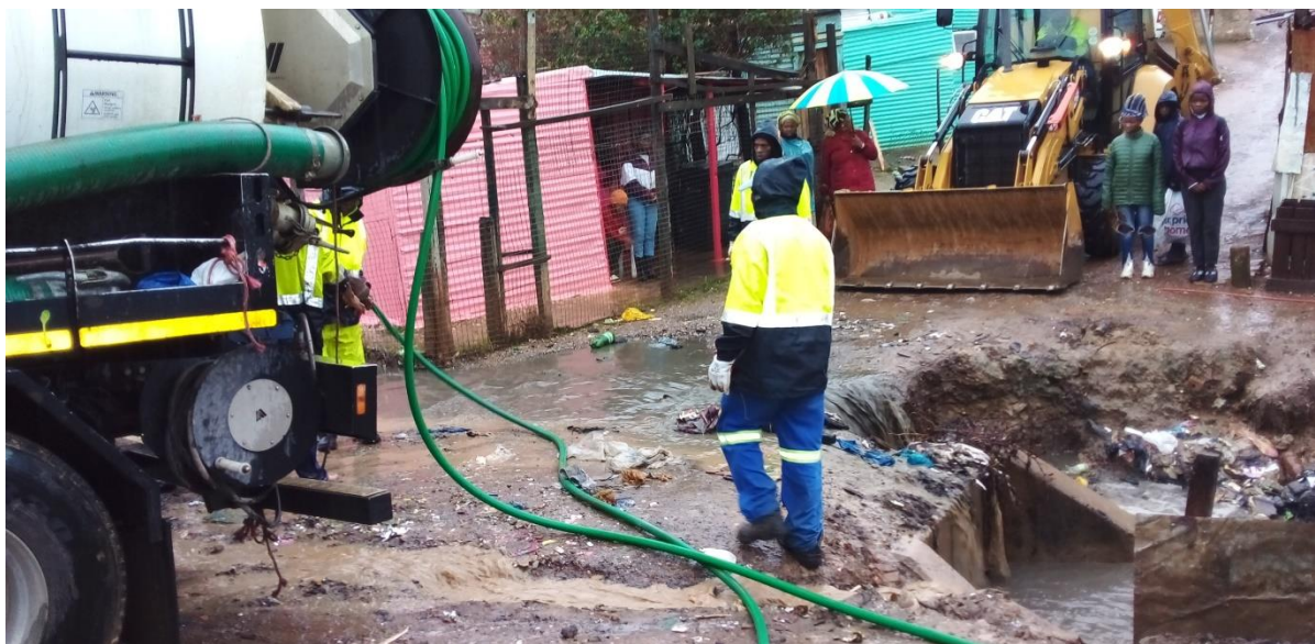
Bridge flooded in Nkanini (Kayamandi) during heavy rain conditions.
