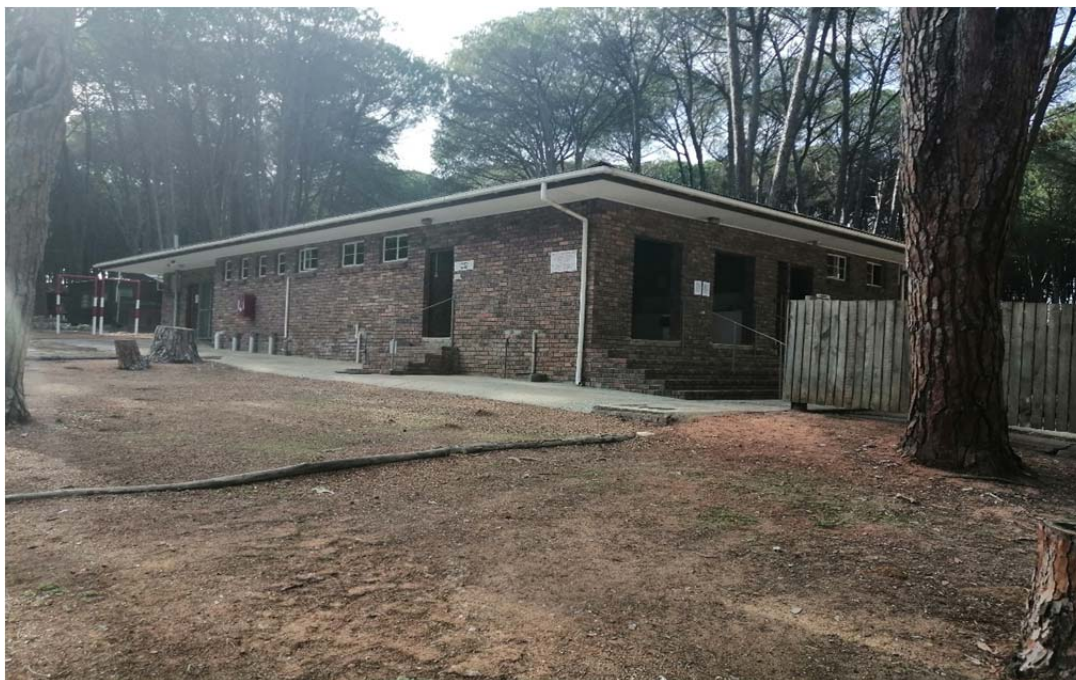
Fig 19: Main ablution facilities
