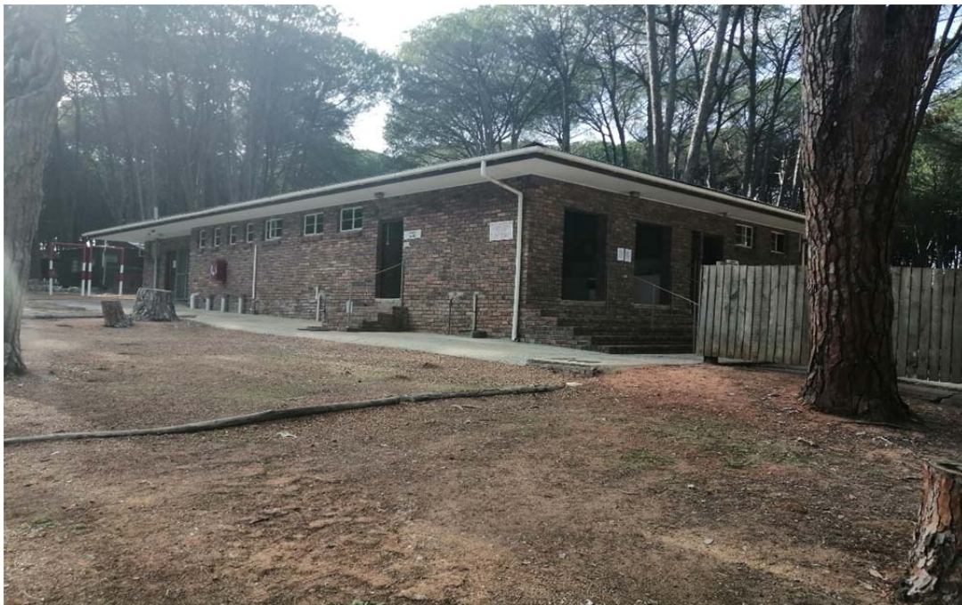
Fig 19: Main ablution facilities
