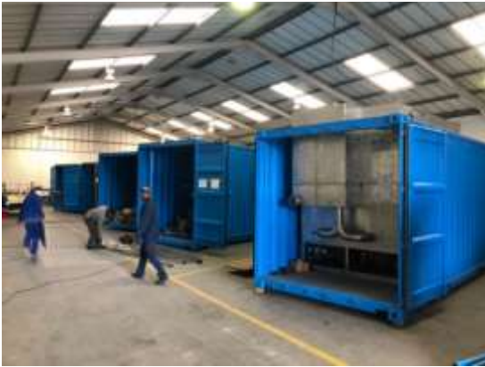
Figure 41: Stellenbosch Containerised WTW being manufactured
