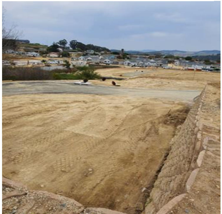
Figure 3:13: Installation of services complete
