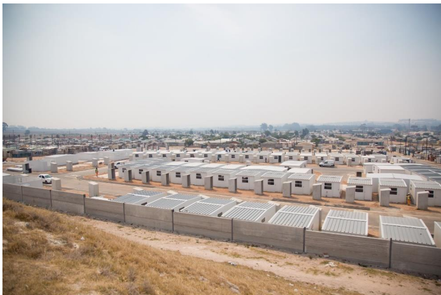
Completion of construction of TRA
