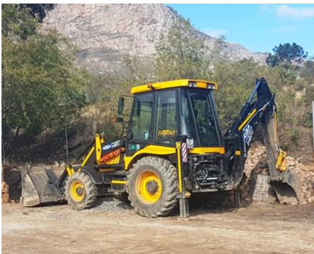
Figure 3:8: Digger loader and front view of 10t tipper truck
