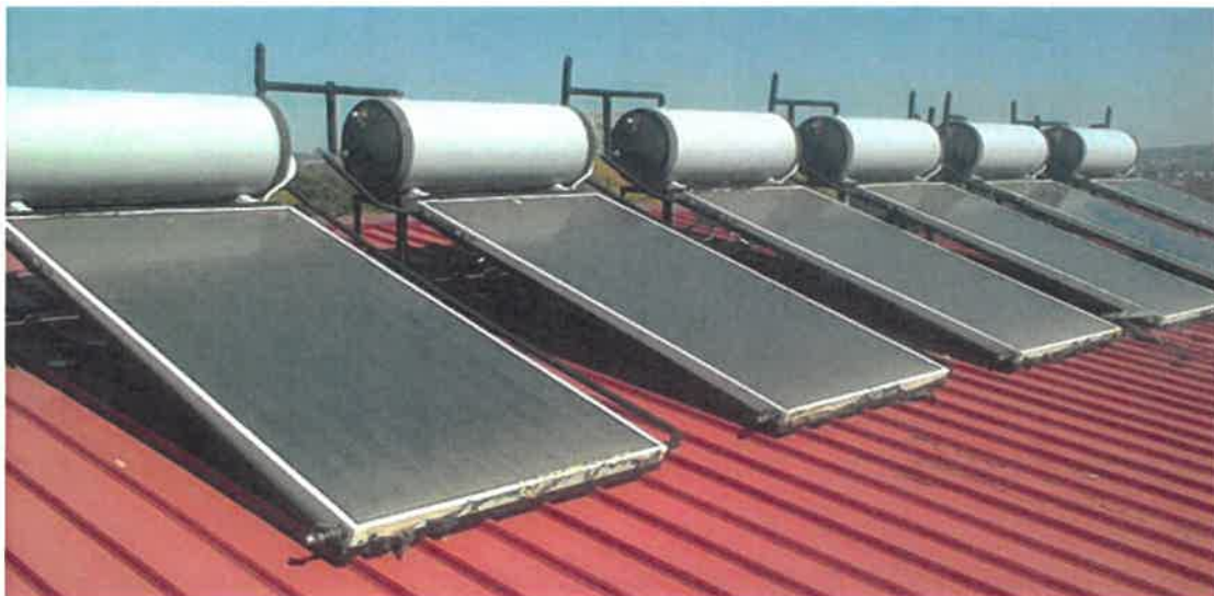
Figure 43: Roof Mounted Solar Geysers
