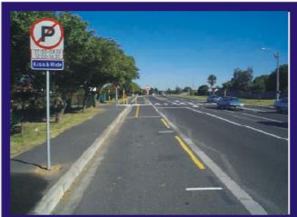
Raised Pedestrian Crossing
