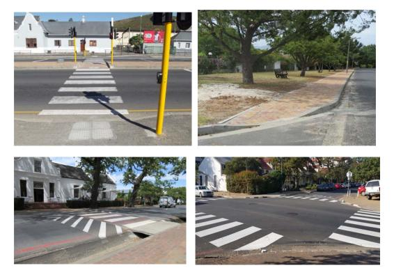
**Project Description:** Sidewalks and dropped curbs, raised pedestrian crossing, tactile paving, audible tactile buttons at pedestrian crossing
