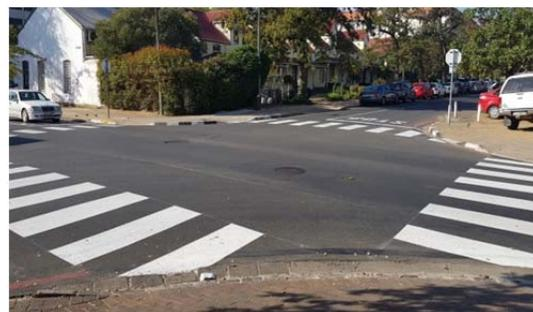
**Project Description:** Sidewalks and dropped curbs, raised pedestrian crossing, tactile paving, audible tactile buttons at pedestrian crossing
