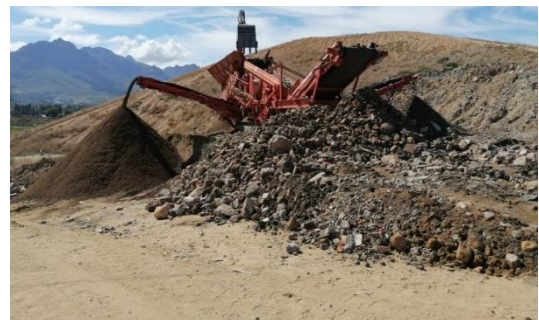
Figure 17: Crushing of builder's rubble done on site
