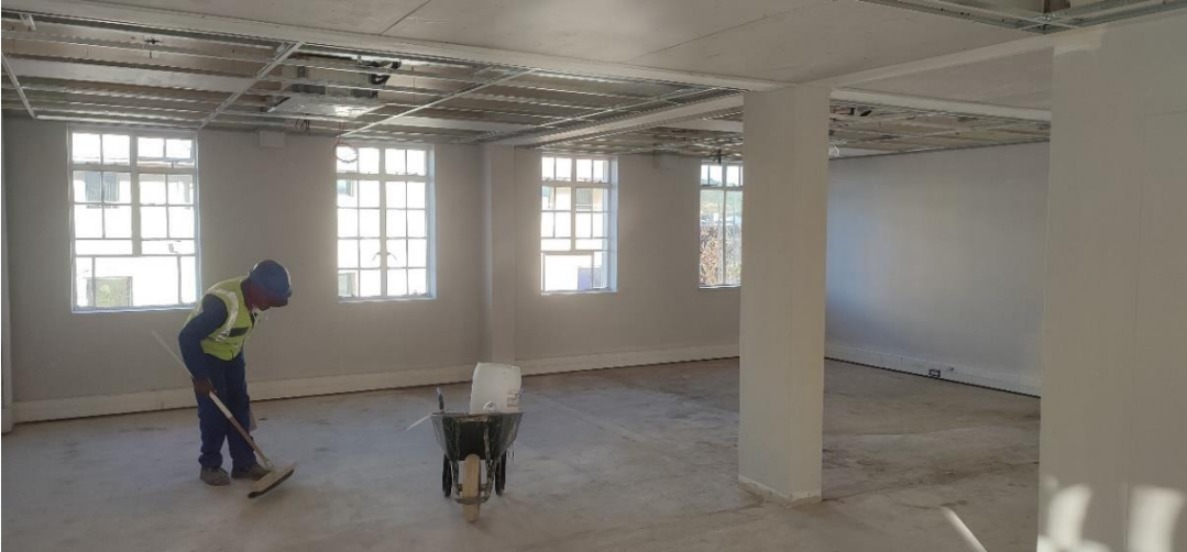
Figure 40: Upgrading of the NPK Building
