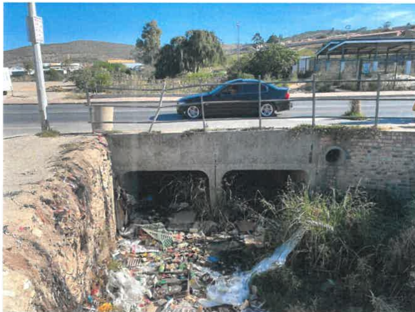
Figure 6: Culvert at George Blake Street
