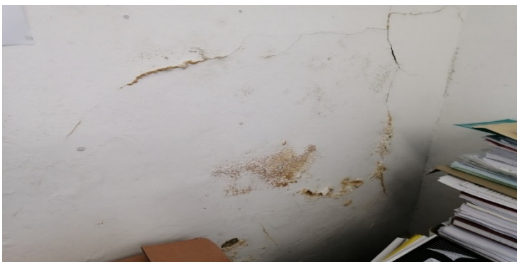
Mould and water damage. Office space – reservoir
