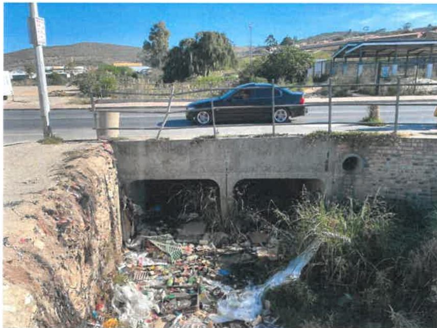
Figure 6: Culvert at George Blake Street
