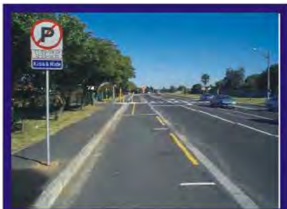
Raised Pedestrian Crossing
