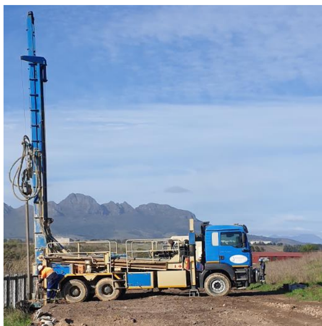
Photo: Drilling of well on-site
