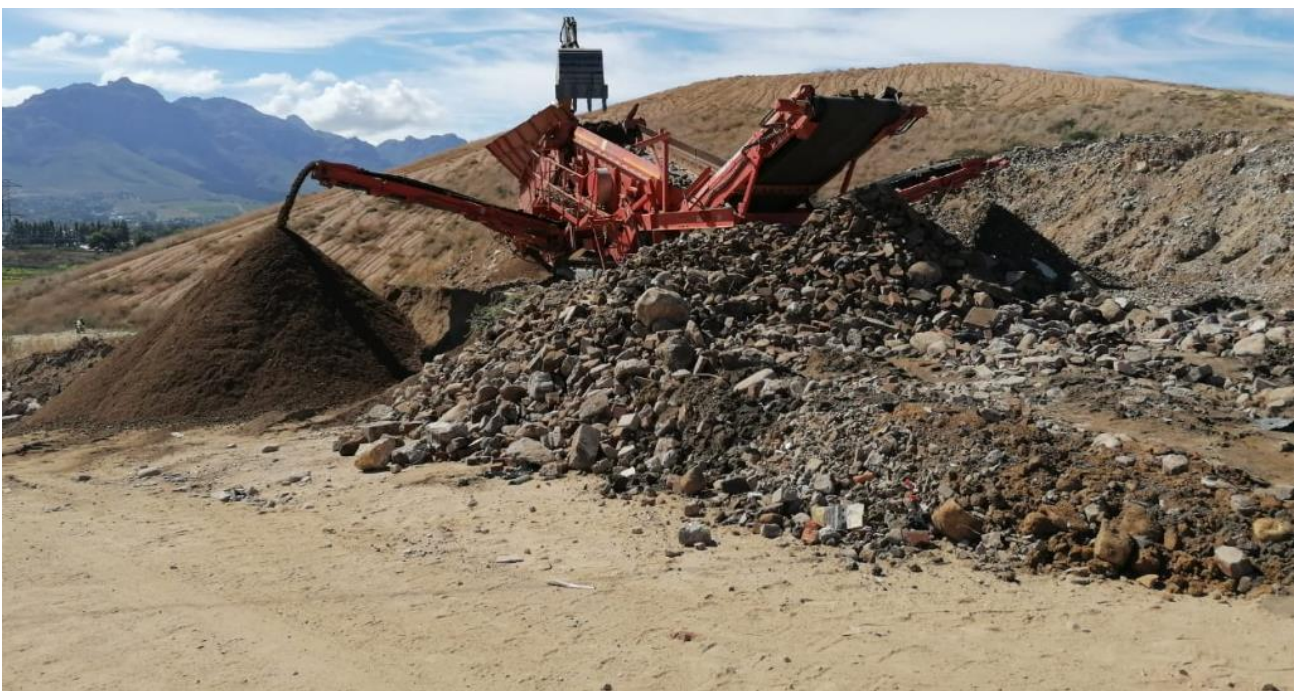
Figure 16: Crushing of builders rubble done on site
