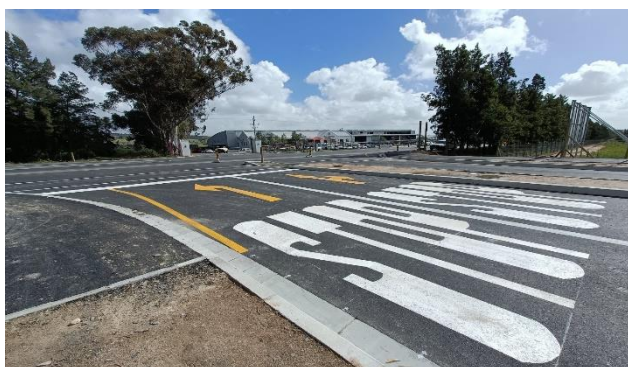
Figure 42: Klapmuts Road intersection Upgrade
