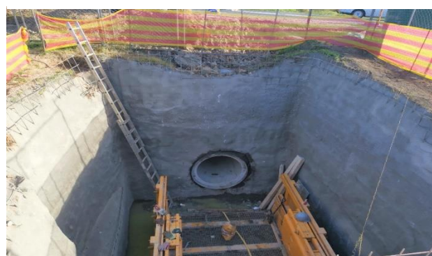
Figure 41: Sewer Crossing Bottelary Road (Devonbosch)
