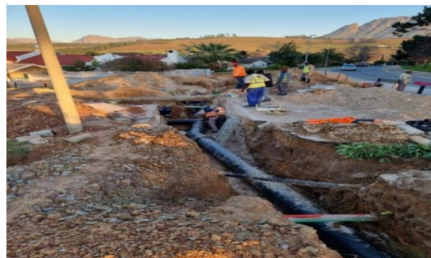
Figure 43: Vlottenburg New Outfall Sewer (Longlands)
