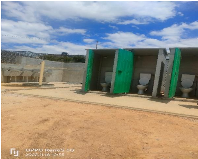
Figure 36: Construction of basic services, Watergang Informal Settlement
