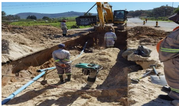
Figure 44: Cloetesville Bulk water upgrade (Voliere)
