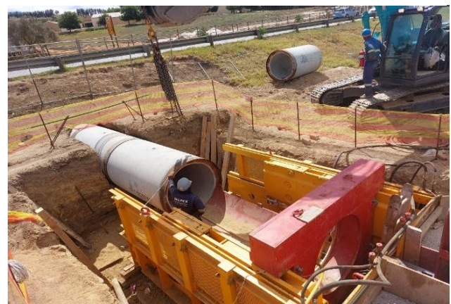
Figure 47: Outfall Sewer upgrade (Newinbosch)
