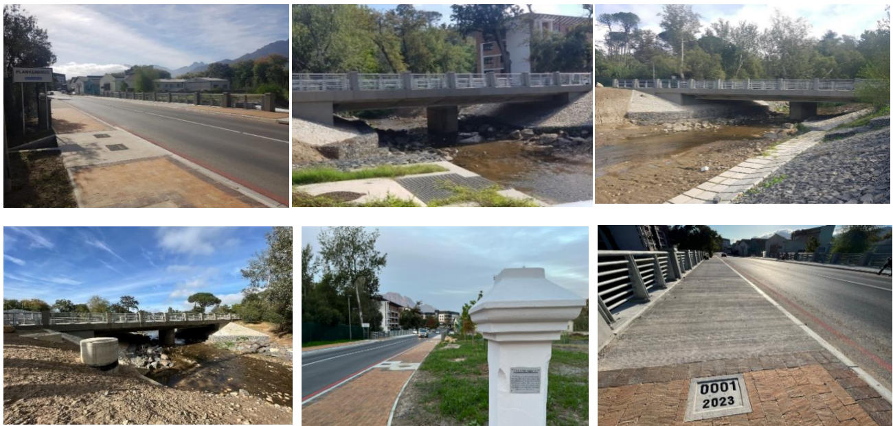
Figure 32: New Bridge constructed
