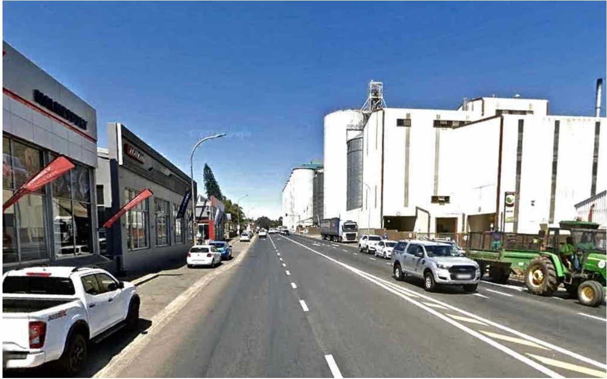
FIGURE 43: The entry into Malmesbury from the west off the N7 along Bokomo Street has been transformed into a 20 th C industrial landscape, largely around the processing and milling of wheat. (Image, Google Earth Street View, August 2022).
