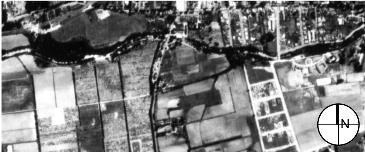
FIGURE 26: 1953: The southern approach into Stellenbosch is still largely unchanged from 1938 and retains a strongly rural character. (SG Historical Aerial Survey Series frame 335_006_06062).
