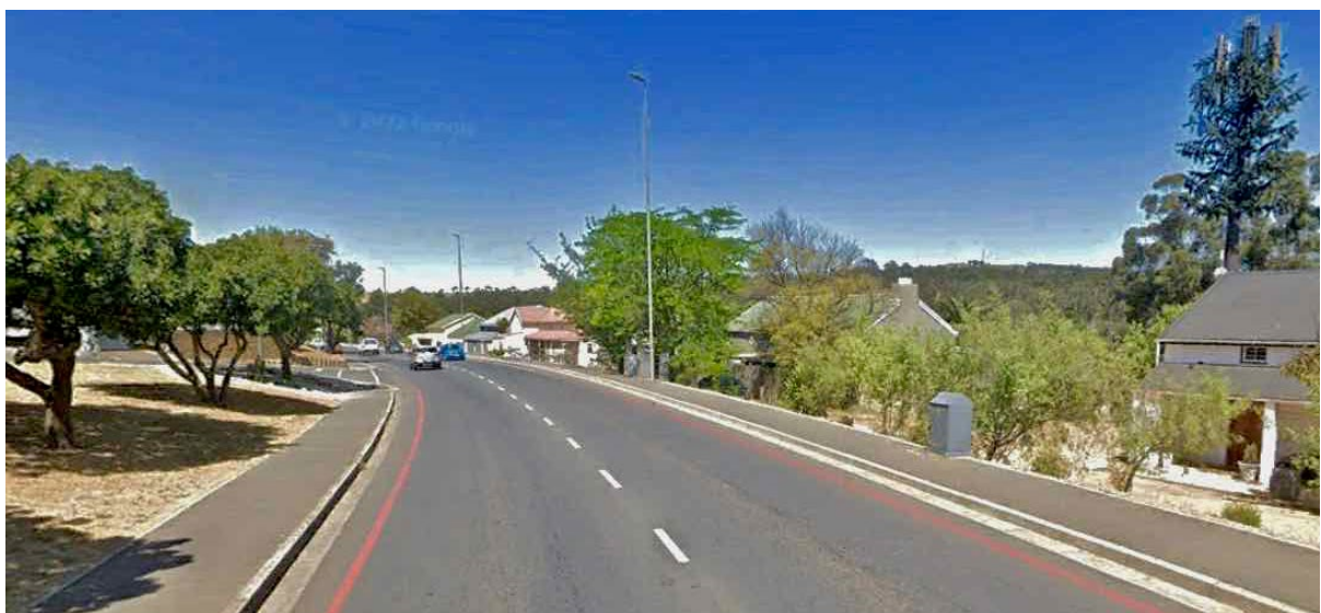
FIGURE 42: Entry along the road from Paarl into Malmesbury. Changes in level and alignment due to 20 th C roadworks have significantly altered the historical integrity of this gateway route which is especially regrettable as a substantial number of late 19 th /early 20 th C dwellings survive along this route. (Image, Google Earth Street View, November 2022).
