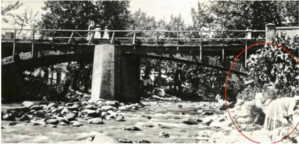
FIGURE 23: The first Victoria Bridge. This structure replaced the Koloniesbrug at some stage between the mid and latter part of the 19 th C. This single arched timber bridge with central support was more substantial than its predecessor. Note the washerwomen on the right (circled) while additional laundry activity can be seen in the background including on the opposite riverbank. The people in this image would have been locals from Roesdorp/Die Bos; the Rhodes Cottages (see vi) below) and dwellings on the north bank of the Eerste River. (From Albertyn, p40 Fig 30. Image from the Stellenbosch Museum: A/b:10b.i.EER).
