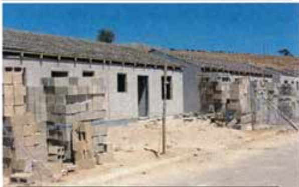
MPAC/Oversight visit Kayamandi housing project
