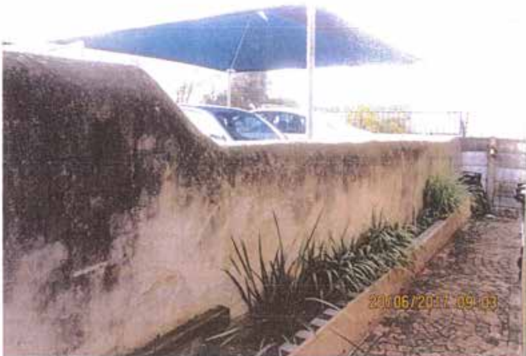
↳ EXISTING WALL BETWEEN ELF 1205 & ELF 13606, STB
