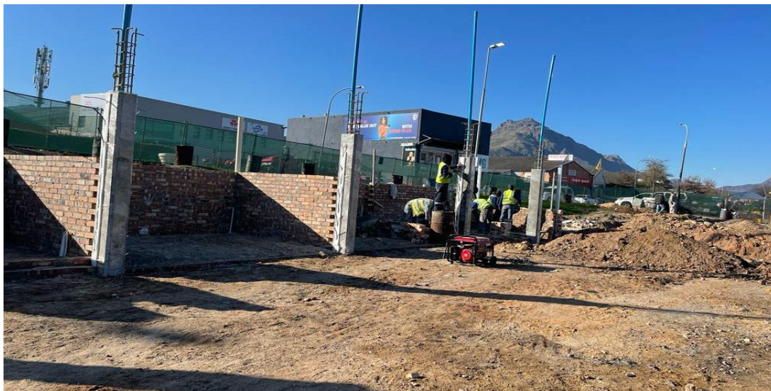
Figure 43: Construction of new taxi rank (Bird Street)
