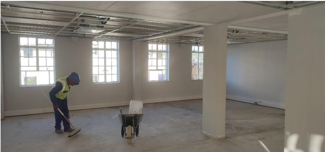
Figure 41: Upgrading of the NPK Building
